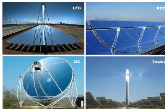
Fig. 1. CSP technologies. LFC Linear Fresnel Collector. PTC Parabolic Through Collector. DC Dish Collector. ST Solar Tower.
