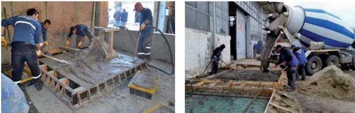
Fig. 2. SUS-CON concretes casting in real production plants
